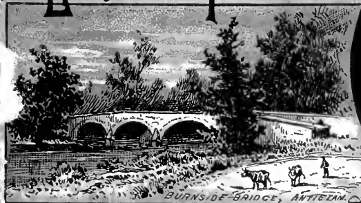
BURNSIDE BRIDGE, ANTWERP, C.
